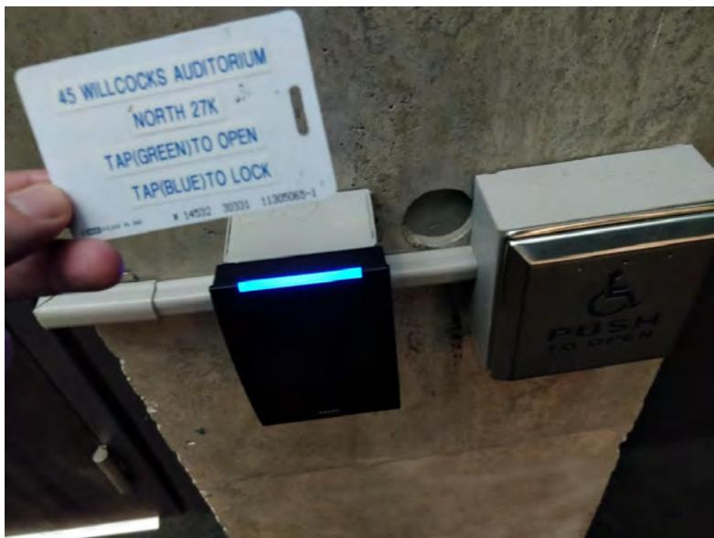
Tap key card "NORTH" to **open Room A** or Tap key card "South" to **open Room B**. Light will turn from **blue** (locked) to **green** (unlocked).
